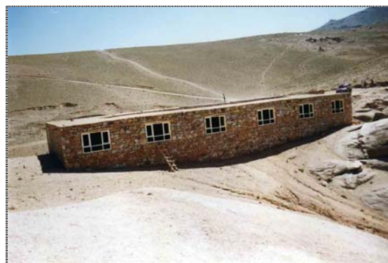
The girls high school was built with stone and cement brought in from a nearby province. It can withstand the severe weather conditions much better than local mud brick buildings.
