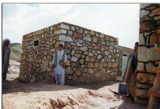
Australian IF representative, Kawa Mobaligh, stands in front of the newly constructed girls high school.
